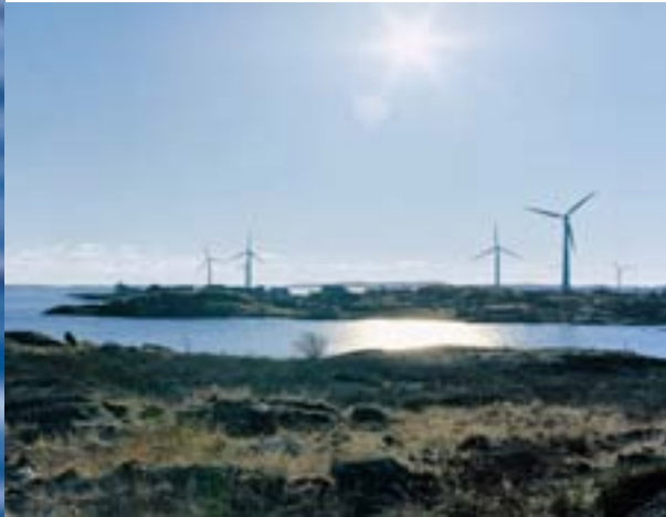
The energy for OPS in Port of Göteborg comes from two wind mills
